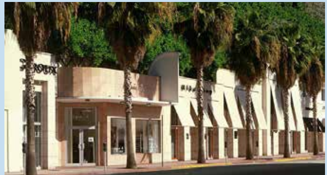
Image 33. Seventh & Collins parking garage.(Source :Arquitectonica)
