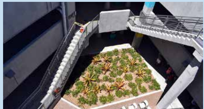
Image 35. St Armands parking garage.(Source: youobserver.com)
